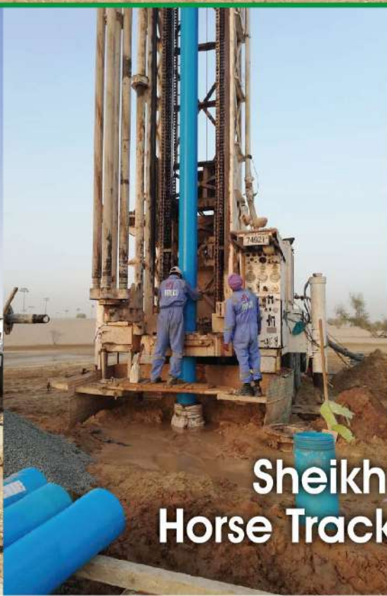
Deep Water Bore Wells Drilling
